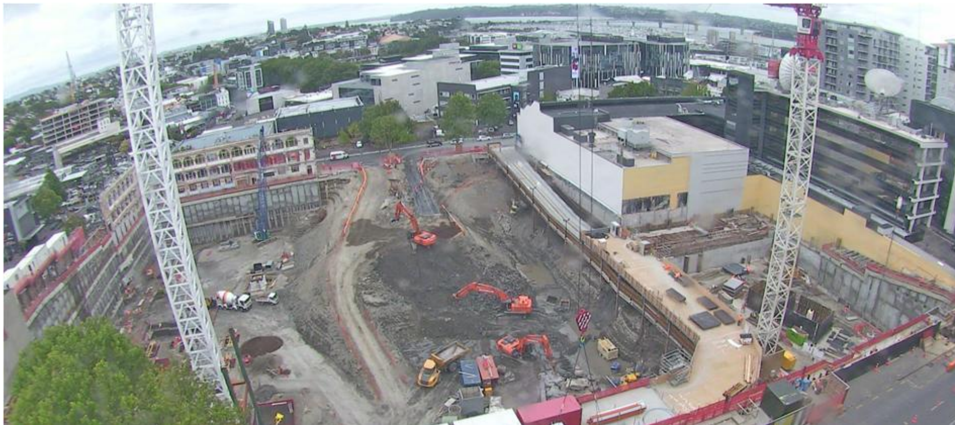
NZICC and Hobson St hotel site as at end of January 2017
